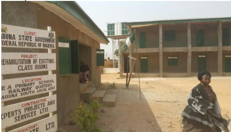
Figure 7: Rehabilitated LEA primary school in Down Quarter (Iliya, 2017)
