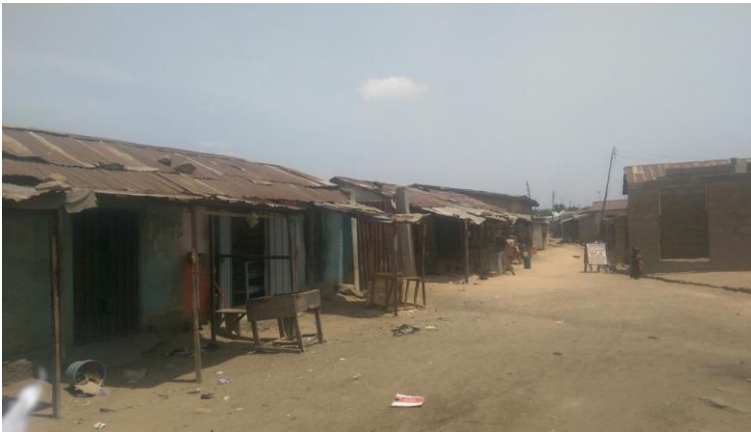
Figure 6: Housing in Down Quarter (Iliya, 2017)
