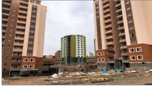
Figure 4: Construction activities pollution in project site (Dhuoki, 2020)
