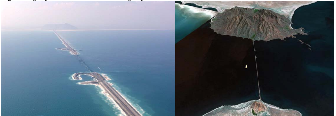
Fig6. Images of The Shabid Kalantari Highway
