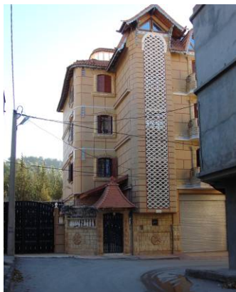
Photo 2: 3 Levels +height (subdivision02); Source: The author (2014)
