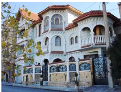
Photo 4: Achieved house, Subdivision 2; Source: The author (2014)
