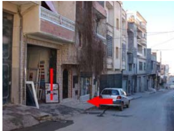
Photo 10: Premise occupied by aluminum joinery, subdivision El Imane; Source: The author (2014)
