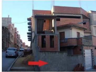
Photo 9: Jardin construit, lotissement El Imane ; Source: The author (2014)
