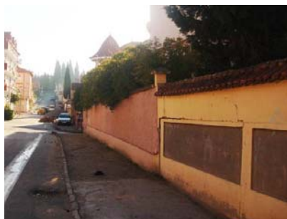
Photo 7 : Fences inside the subdivision 01; Source: The author (2014)
