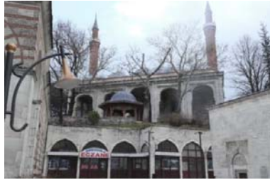
Figure 37. Yuldırım Bayezîd Mosque today (Authors' archive, 2017)
