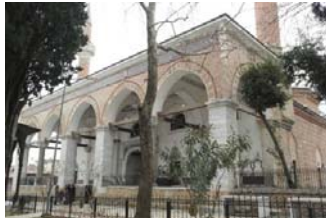
Figure 57. Front facade of Muradiye Mosque (Authors' archive, 2017)
