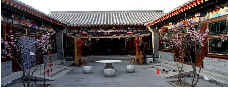
Pic. 1: Han architecture with bricks and tiles
