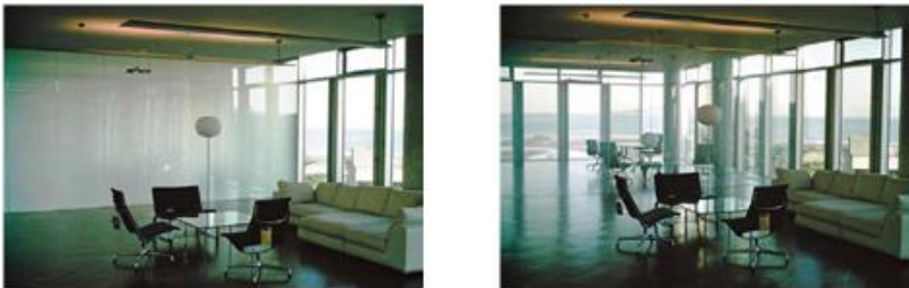
Figure 7: switchable glass enabling visual contact and natural daylighting (source: Fox, M., & Kemp, M. (2009)
