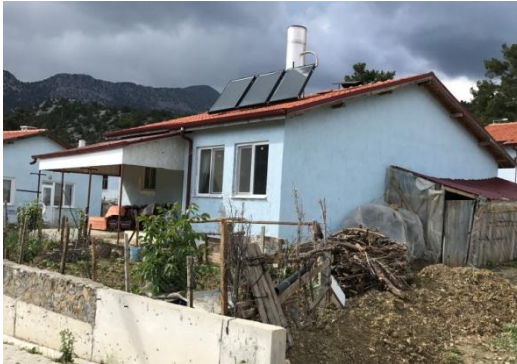
Figure 8. House with the frames replaced and window, terrace, lean-to-roof and woodshed added
